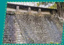
C 砌石擋土牆 A Masonry Retaining Wall
