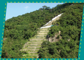
B 美化山泥傾瀉殘痕 Landscaping a Landslide Scar
